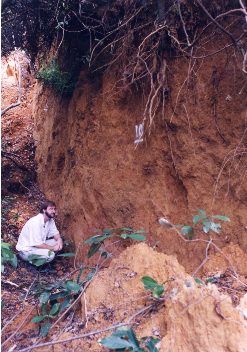
Plate 8 - Main Scarp, Vertical Displacement at this Point is 3.8 m (Plate Location Shown on Drawing EG503) (Taken on 26/9/97)
