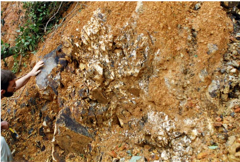
Plate 30 - Rhyolite Dyke Exposed in Landslide Scar 4 - Note Very Closely Spaced Joints with White Kaolin Infill (Plate Location Shown on Drawing EG503) (Taken on 7/7/97)
