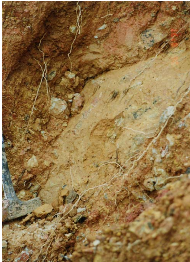
Plate 24 - Surface of Rupture Through Intact Saprolite Exposed in Landslide Scar 4A - Note Sharp Interface Between Recent Debris and Surface of Rupture (Plate Location Shown on Drawing EG503) (Taken on 27/8/97) EG 97/109/15
