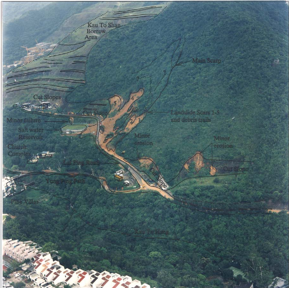
Plate 1 - Oblique Aerial View of Lai Ping Road Landslide Site from the South, Annotated to Show Landslide Scars 1-5, the Approximate Location of the Main Scarp, the Extent of the Debris, Locations of other Minor Failures, the Kau To Shan Borrow Area, the Church Complex and Other Structures (Taken on 4/7/97)
