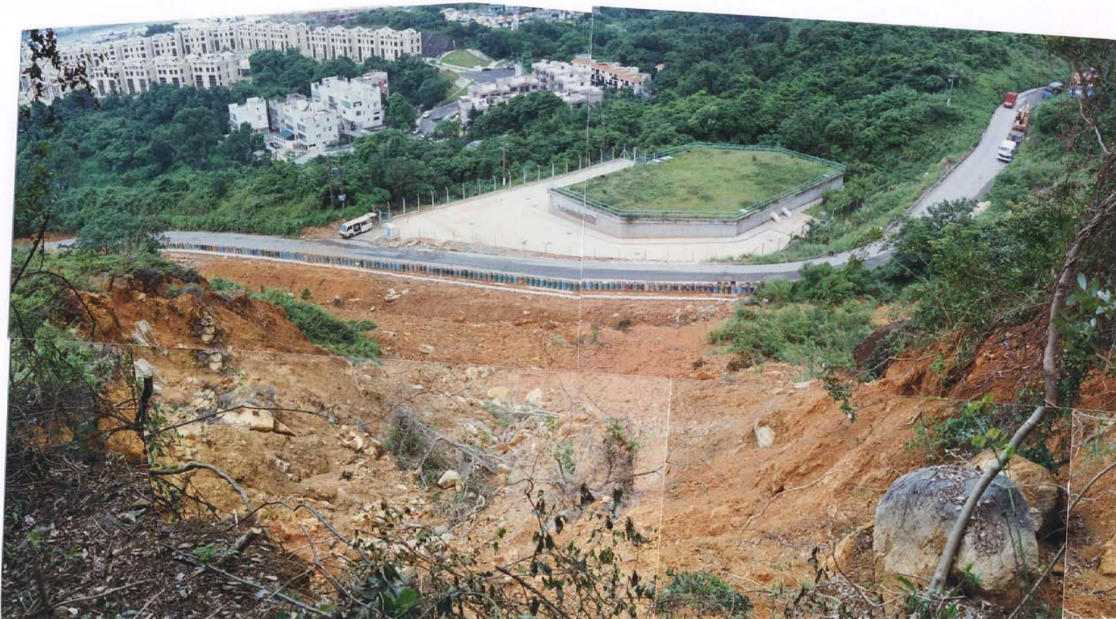
Plate 3 - Covered Surface Reservoir, Lai Ping Road and Pine Villas in the Valley Base - Viewed from the Crest of Landslide Scar 4A, Looking South (Plate Location Shown on Drawing EG503) (Taken 29/7/97)
