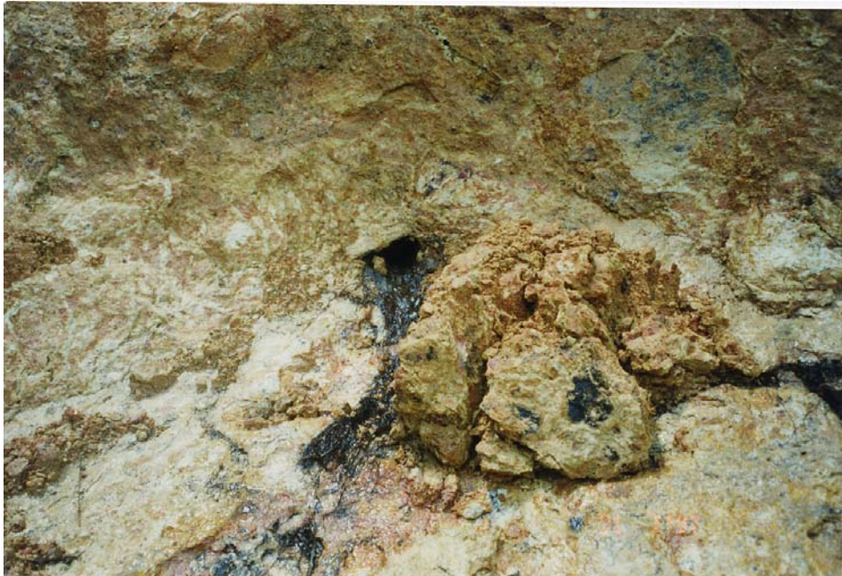
Plate 29 - Small 40 mm Diameter Soil Pipes at the Old Colluvium-Saprolite Interface Exposed in Landslide Scar 5 (Plate Location Shown on Drawing EG503) (Taken on 21/7/97)
