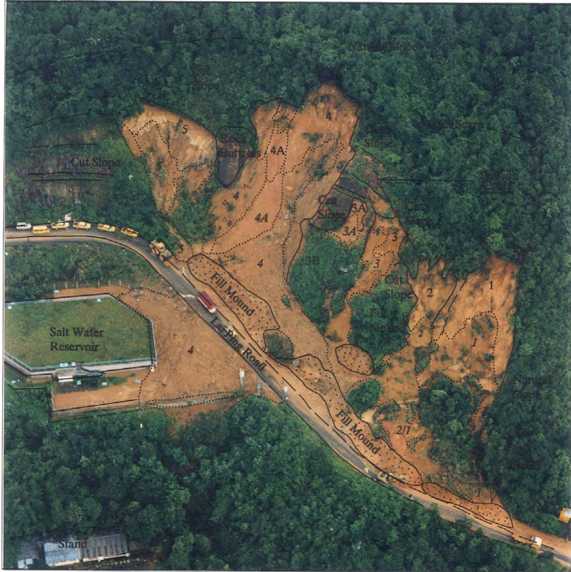
Plate 2 - Oblique Aerial View of Lai Ping Road Landslide from the South-West, Annotated to Show Landslide Scars 1-5 and Associated Debris and Part of the Main Scarp (Taken on 4/7/97)
