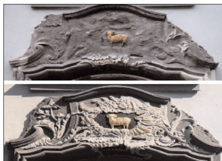
Figure 8. Effect of conservation treatments using calcinogenic bacteria. (Courtesy of Dr Franz Möll, ars restauro, Germany)
