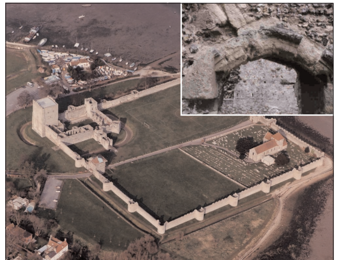
Figure 1. Portchester Castle: a historic monument suffering stone biodeterioration. Figure 2 (inset). Stone decay and crusts on decorative arches at Portchester Castle.
