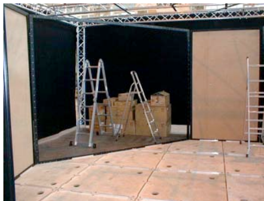
FIGURE 3: The interactive floor in construction
