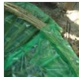
Making seals in the plastic liner
