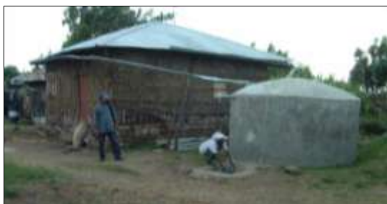
Figure 2: unsustainable DRWH structure.
