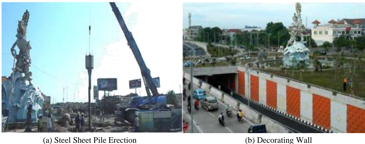
Figure 1 Steel Sheet Pile Erection and Decorating Wall
