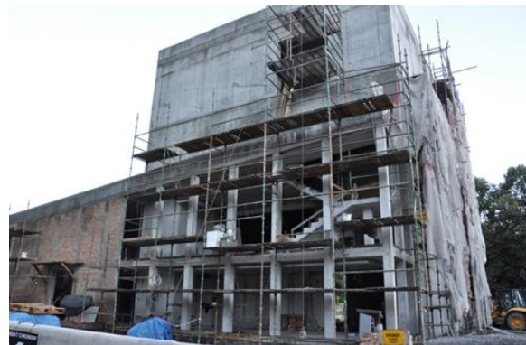
Figure 7. Construction of the I3DVL building (September 2, 2013).
