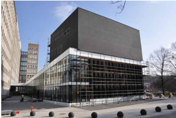
Figure 8. I3DVL building almost ready (March 7, 2014).
