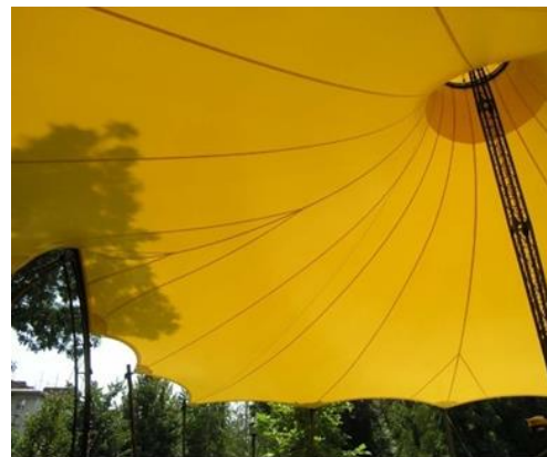
Figure 14. The seams on the cone tent
