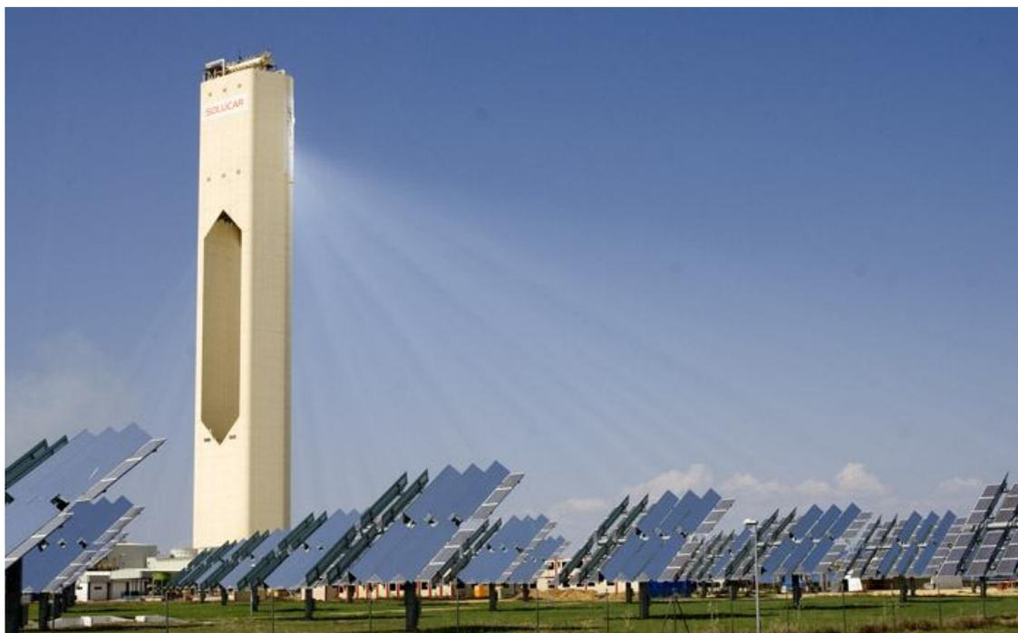
Figure 3 – Solar power tower
