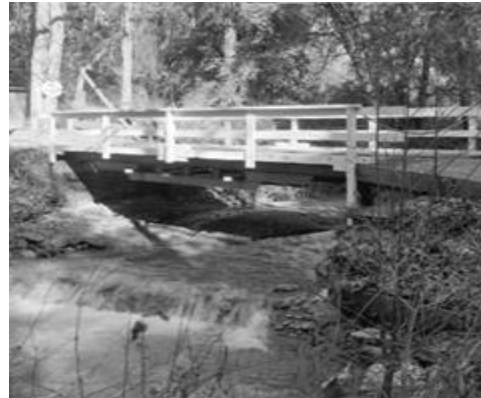
Figure 2. Walk bridge image
