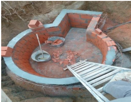
Figure 7. Base Construction of Digester
