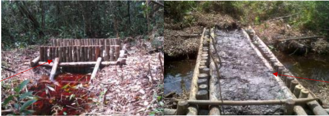
Figure 8. Tabat made by the Kalimantan Dayak Indigenous people (left). The completed tabat (block) was planted with an endemic plant (right). Images can be seen at https://orangutan.or.id/id/mawas-peatland-rehabilitation-program
