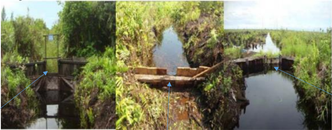
Figure 7. Simple floodgates to raise the surface of the water so that the foliage is always wet. Pictures can be seen in book of “Lahan gambut Indonesia, Pembentukan, Karakteristik dan mendukung ketahanan pangan”, revised edition, Balitbangtan, Ministry of Agriculture. 2016. Chapter 6 Page 142
