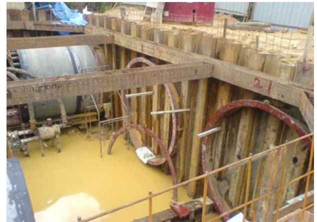
Figure 6 Three 3 m drainage microtunnels to divert the river flow (Hall, 2010)
