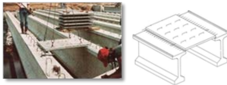
Figure 1. Precast panel deck slab
