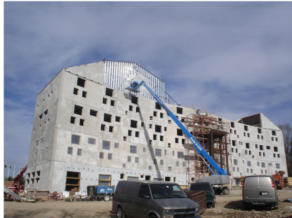
Figure 3: Pre-cast concrete structure. Source: (Author 2006)
