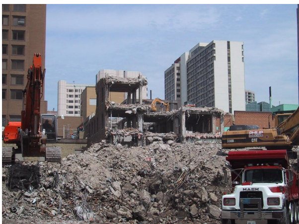
Figure 5. Demolition is more often the outcome of obsolescence rather than physical deterioration.
