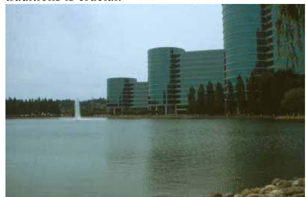
Figure 6. Oracle Campus, Silicon Valley, CA (1989 – 1998, Architect: Mitchell Schwarz, Photo by Umut Toker).
