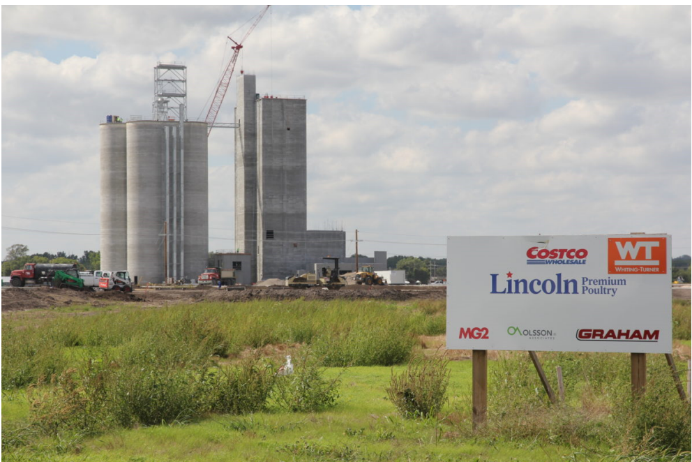
Figure 4: Fremont’s new poultry processing facility. (Photo courtesy of Twilight Greenaway Animal Welfare, Rural Environment and Agriculture Project.)
