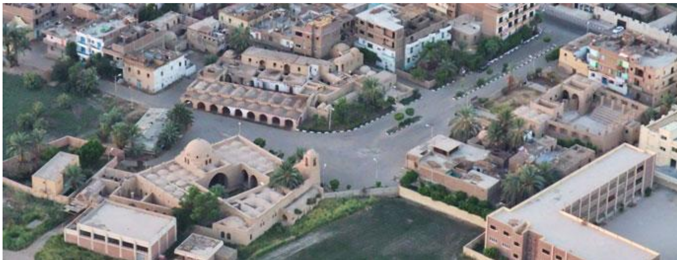
Safeguarding project of Hassan Fathy's New Gournah Village. New Gournah Village is located in Luxor on the West Bank of the Nile River, within the World Heritage property of Ancient Thebes in Egypt. The Village was designed and built between 1946 and 1952 by the famous Egyptian architect Hassan Fathy (1900-1989). http://whc.unesco.org/en/activities/637/
