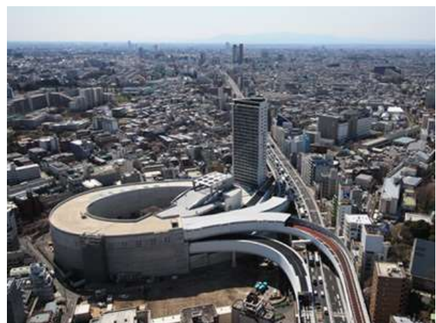
Figure 7. A bird's-eye view of a junction connecting viaduct with underground expressway in Tokyo (Metropolitan Expressway Company Limited. HP, 2011)
