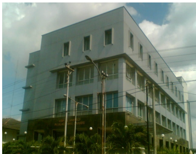
Figure 1. The building of IRD RSUP Dr. Sardjito Yogyakarta
