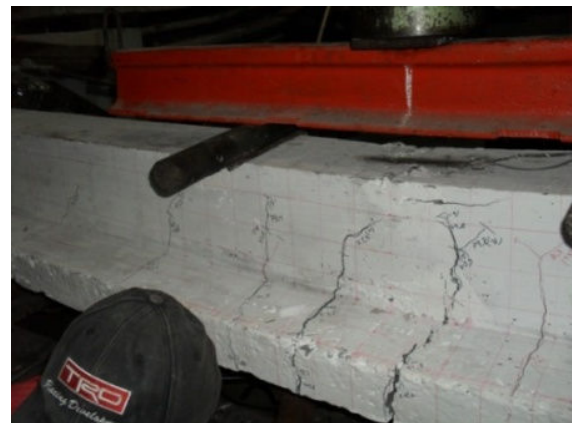
Figure 11. The pattern of crack in the reinforced beam of type 1
