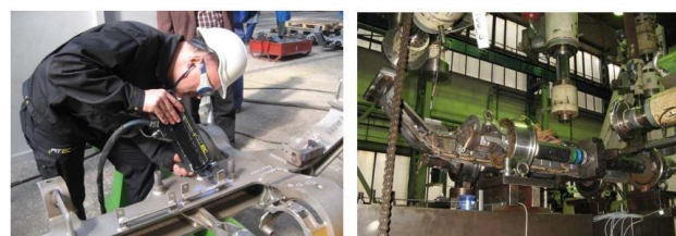
Fig. 20: Weld treatment using HFMI/PIT on train bogie and test facility
