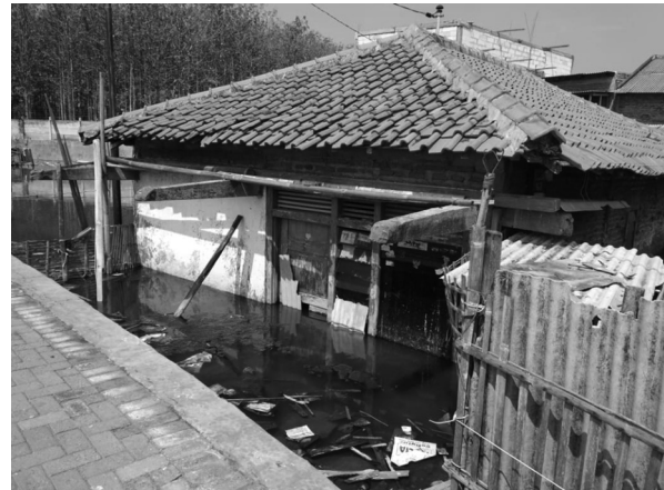
Picture 1. Houses Submerged by Tidal Flood in Terboyo Kulon
