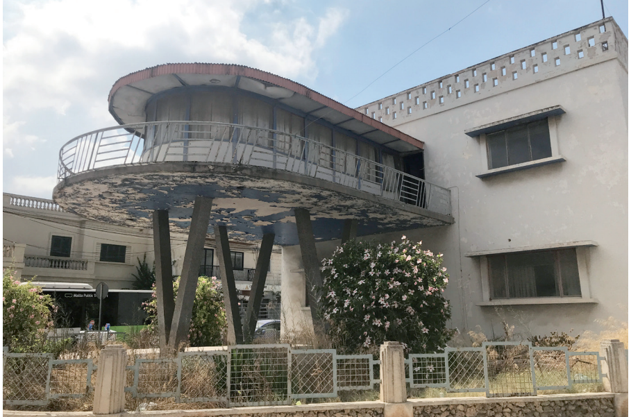
Fig. 1: Photograph of a twentieth century house at the crossroad between Naxxar Road and Francis Xerri Street in B'Kara. (Photo credit: Sandra Mifsud Bonnici)
