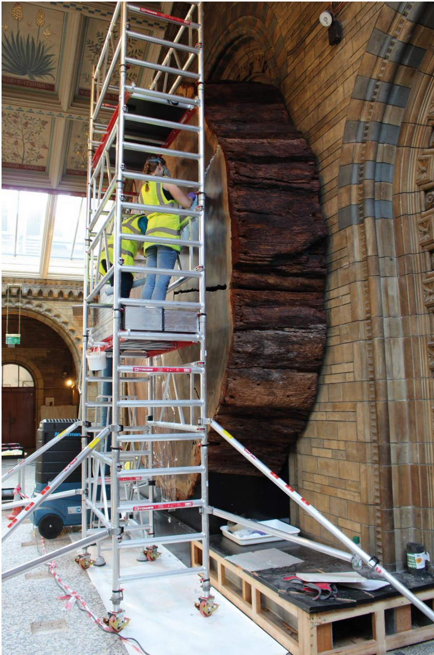
Fig. 4 Working on the scaffolding tower within the gallery.
