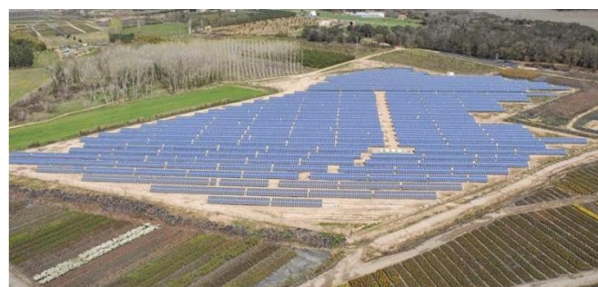
Figure. 1 photovoltaic farm in Spain
