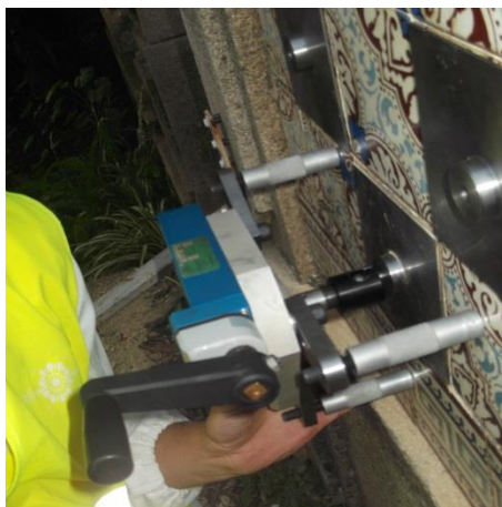
Figure 10 - Adhesion strength test in old facade
