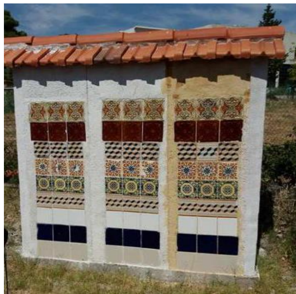
Figure 10 -Exterior wall (south) after 365 curing time days
