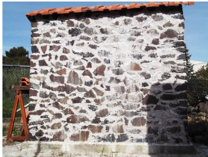
Figure 5 - Exterior wall before tile applications (South facade)
