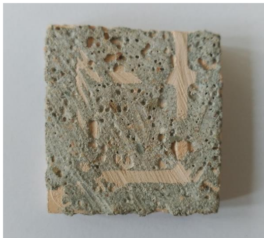
Figure 7 – PC mortar removal
