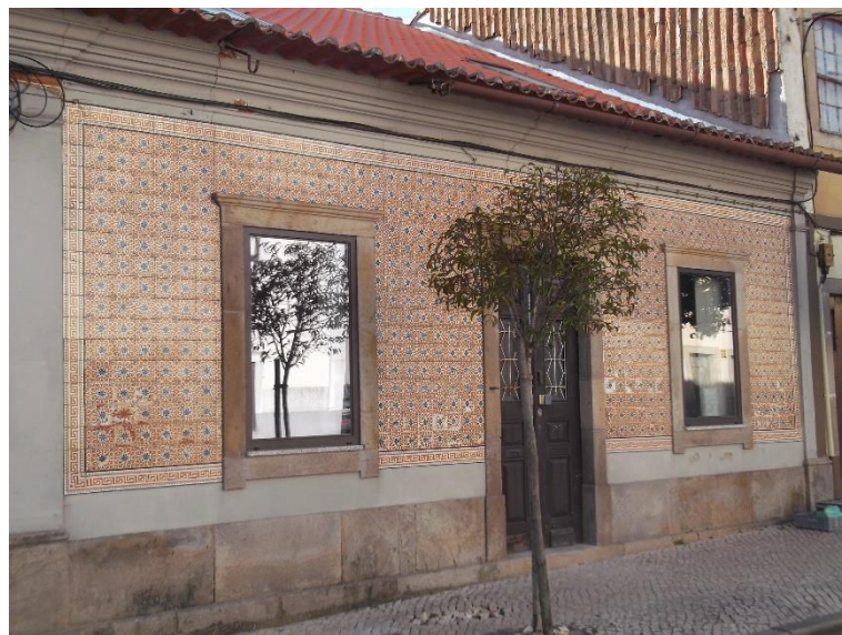
Figure 1 - Exterior building tiled facade
