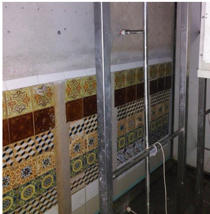
Figure 6 - Interior of climatic chamber during rain simulation cycles
