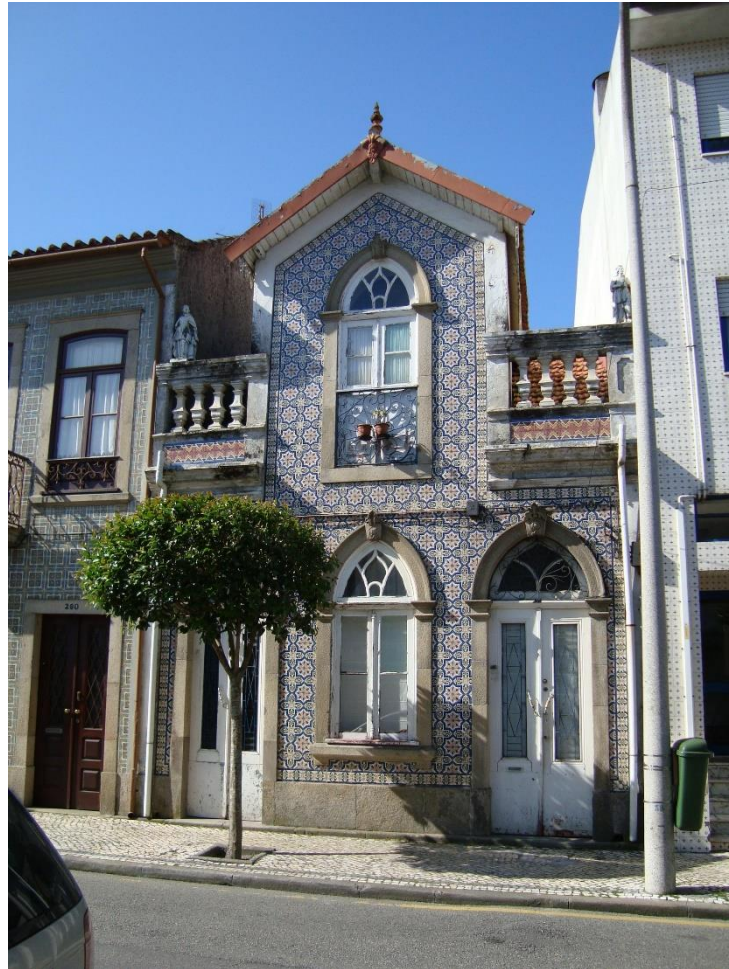
Figure 1 - Tiled facade in Ovar city
