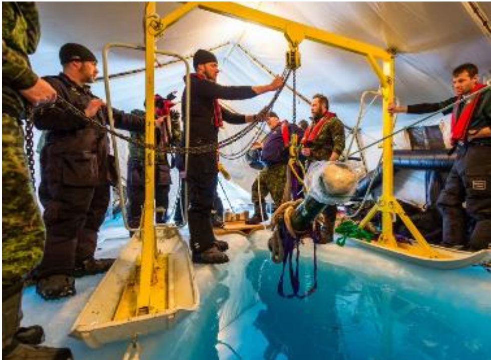
Figure 5.21: 'One of the HMS Erebus 's cannons, recovered through a hole cut out of nearly two metres of Arctic sea ice, is hoisted up by the combined Parks Canada and Fleet Diving Unit Atlantic team.'
