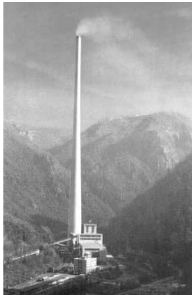
Fig. 2. – The Trbovlje Thermal Power Plant with a 360 m stack.
