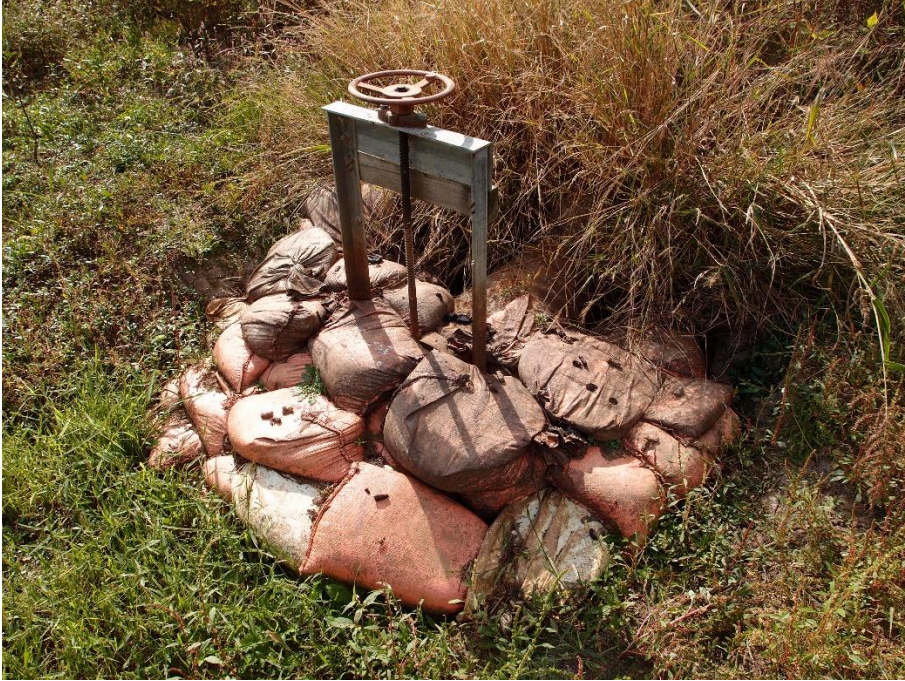
Figure 21. Water control structure that has not been maintained on an easement in Greene County.
