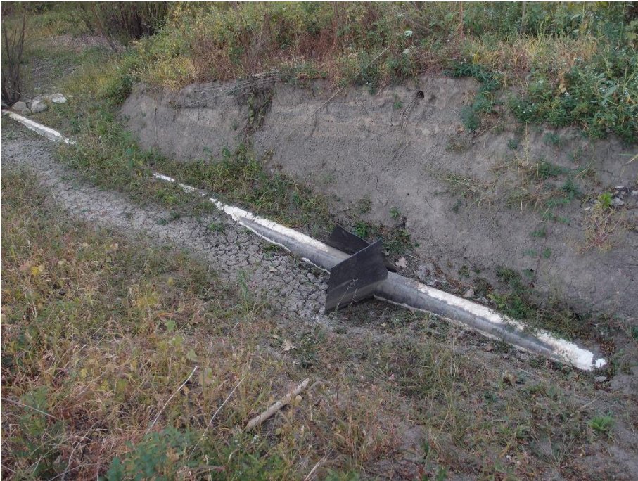
Figure 7. Exposed drain pipe due to soil erosion on an easement in Greene County.
