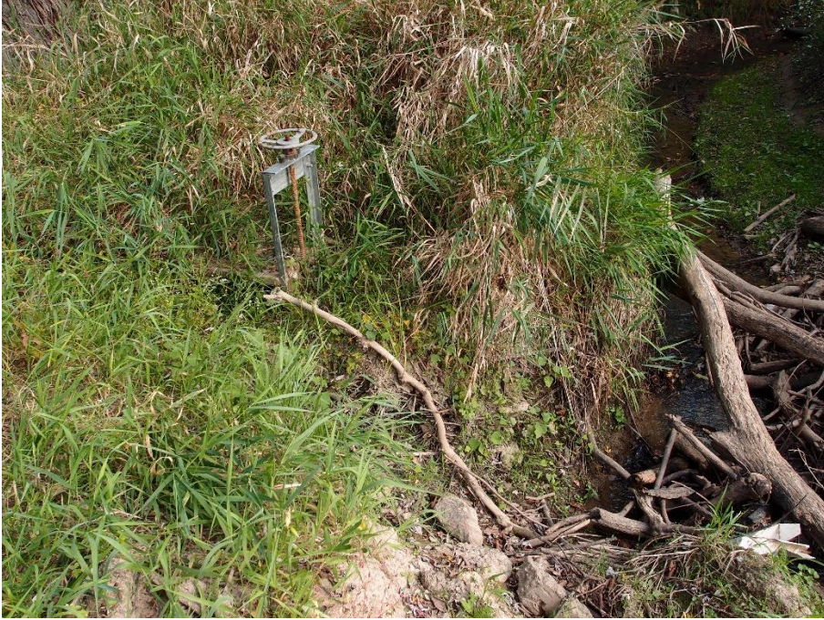
Figure 19. Screw gate that has been made inoperable near an easement in Madison County.
