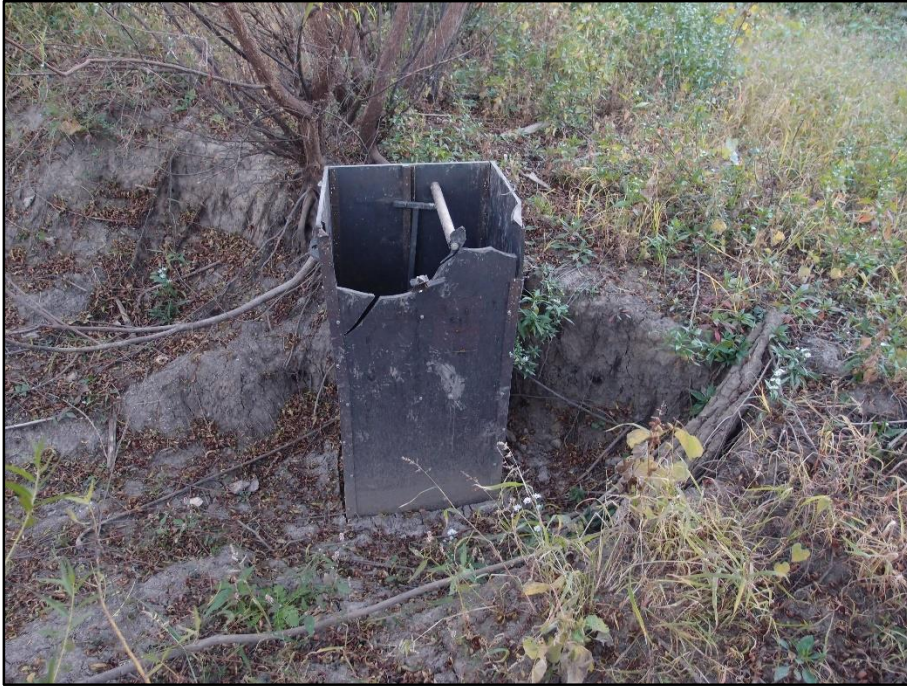
Figure 7. Exposed drain pipe due to soil erosion on an easement in Greene County.
