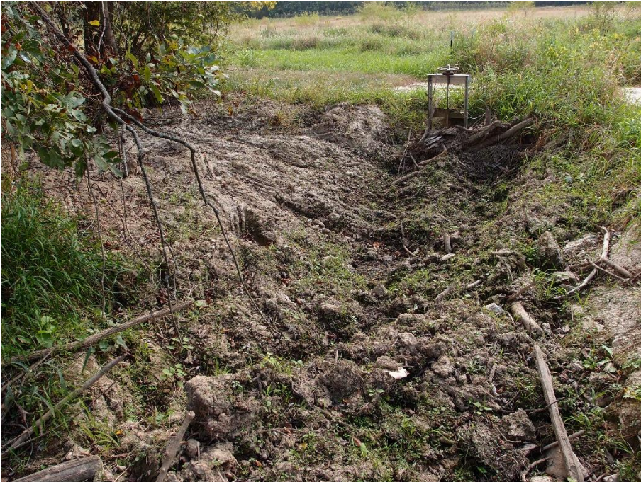
Figure 19. Screw gate that has been made inoperable near an easement in Madison County.
