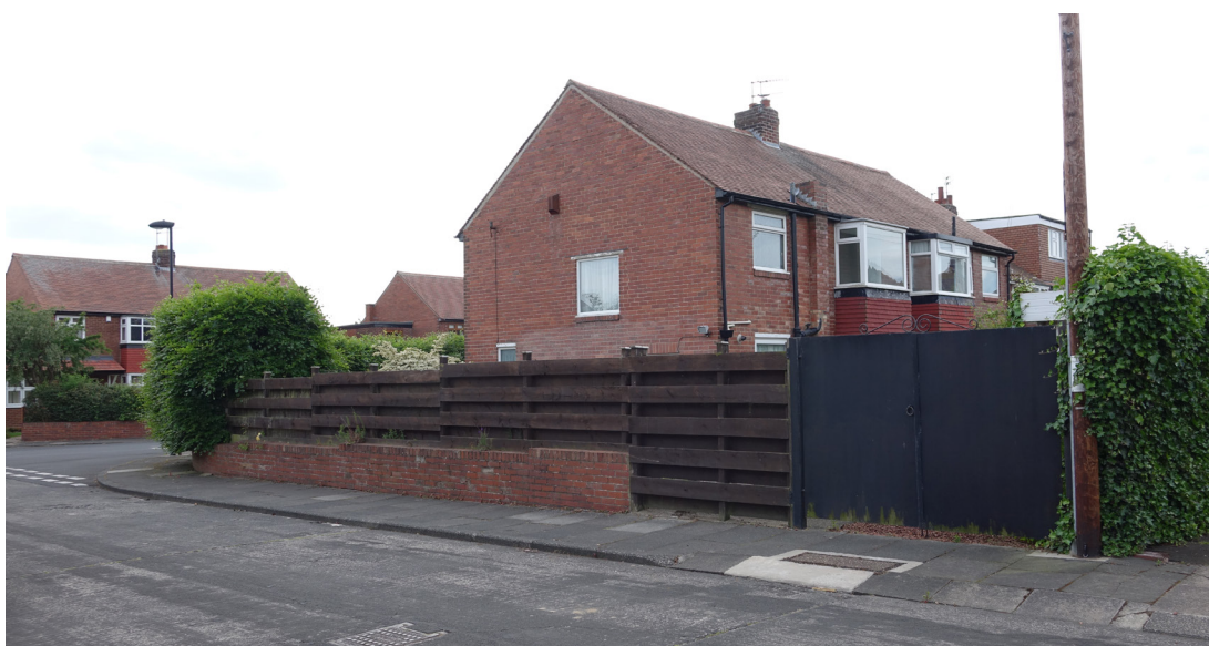
Figure 5.16 - Visually impermeable side interface between the end semi-detached house and the street on Thornfield Road in Newcastle (Photograph by Author, taken on 28.09.2019).
