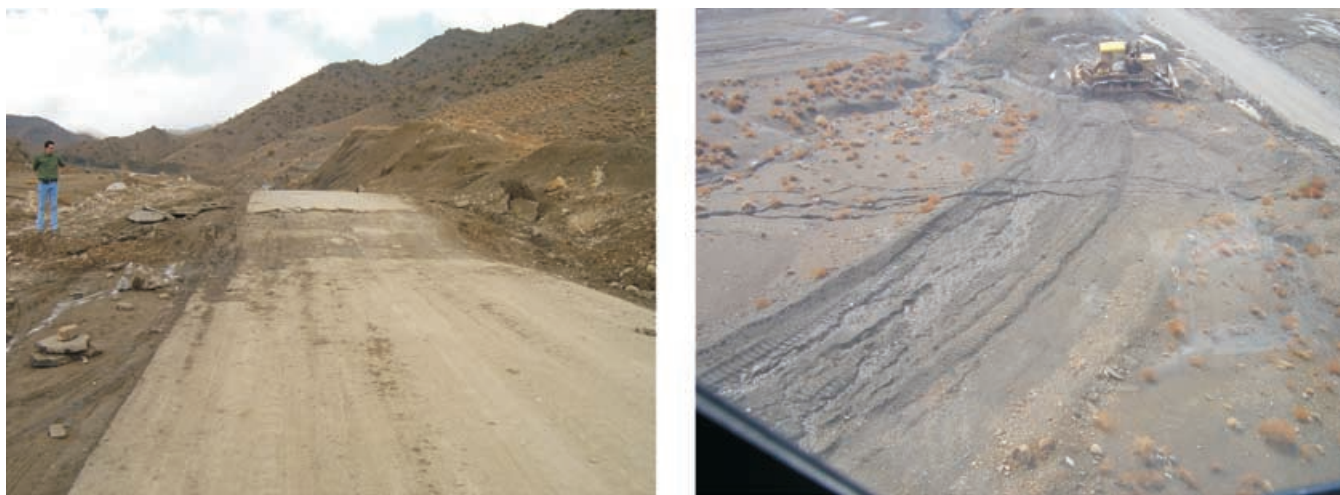
Figure 4. (a) View north of the coseismic rupture cutting the Darbidkhun-Hotkan road (see Fig. 2a) at 30^{\circ}46.993'N 56^{\circ}49.075'E . This picture was taken 1 day after the earthquake, by which time the scarp had been smoothed by bulldozer. The vertical offset is 105 cm. (b) View S from the air of the same locality as (a) on the eastern side of the road, showing a series of parallel open fissures caused by the collapse of the overhanging hanging wall.
