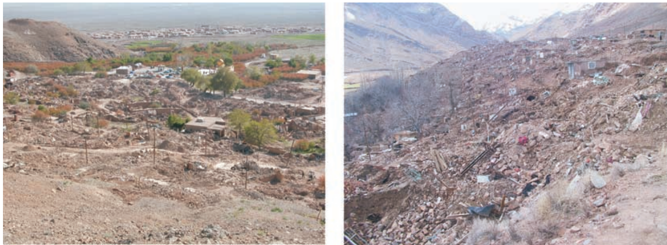
Figure 7. (a) View west over Dahuiyeh. Old Dahuiyeh is almost totally destroyed in the foreground. In the background, on the Zarand plain, is the more modern settlement of new Dahuiyeh, resettled before the earthquake and considerably less damaged. (b) View west along the ridge of Hotkan. The village is completely destroyed, with hardly a building left standing. Only a few door and window frames remain identifiable.
