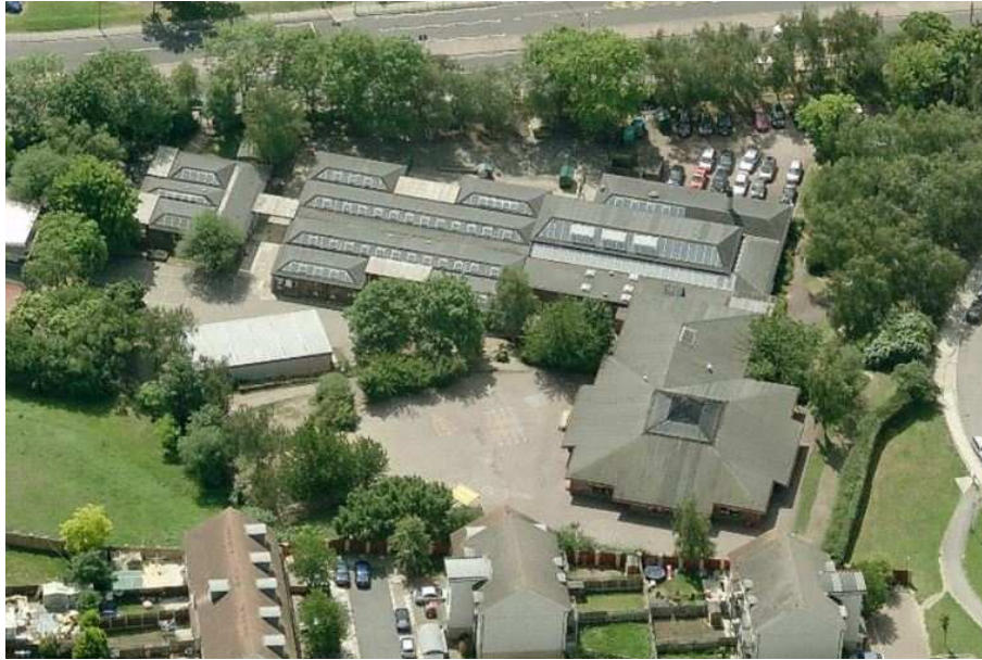
Figure 7.14 Satellite image of a school with roof lights
