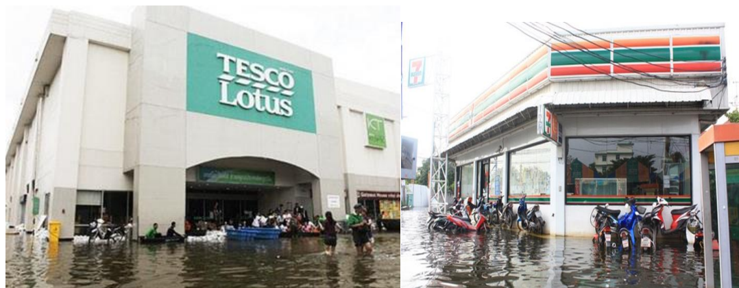
Photo 1.1. Flooding the supermarket and convenience store
