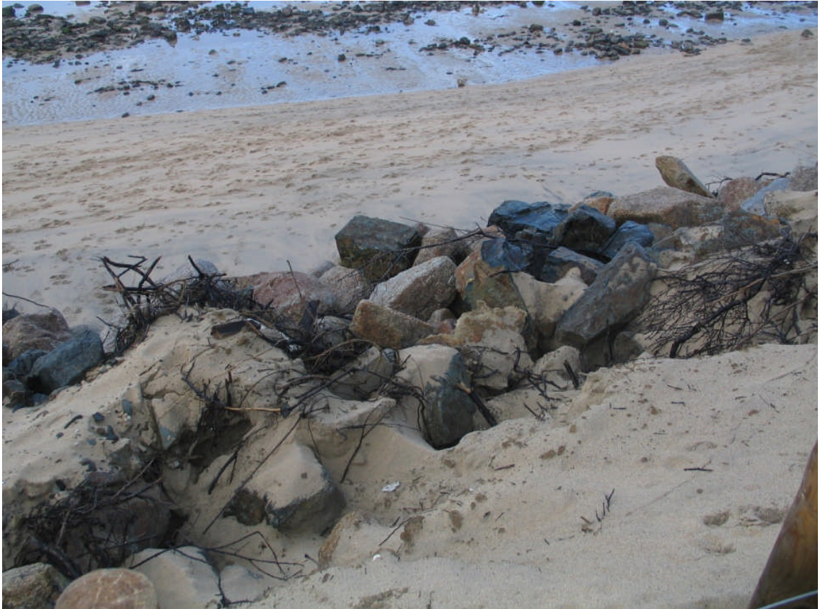
Figure 3.11 Some rocks fragments and stones left at Black Cliff by some residents or concerned organisations in a bid to check erosion at the beach (Field picture, 25/10/2011).
