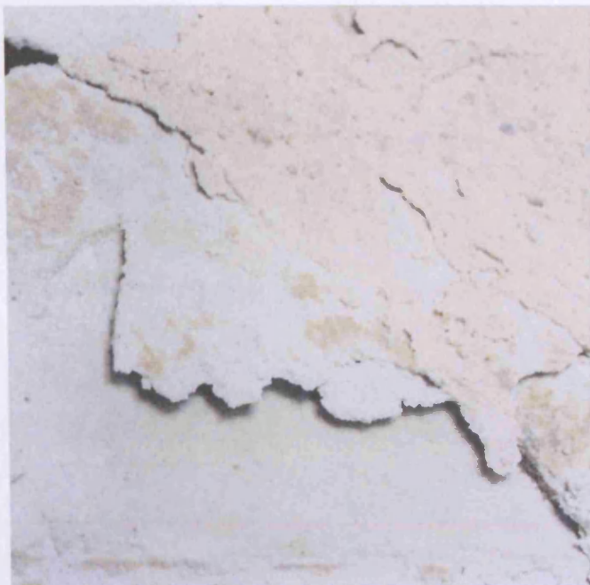
Figure 17 Multiple layers detachments
