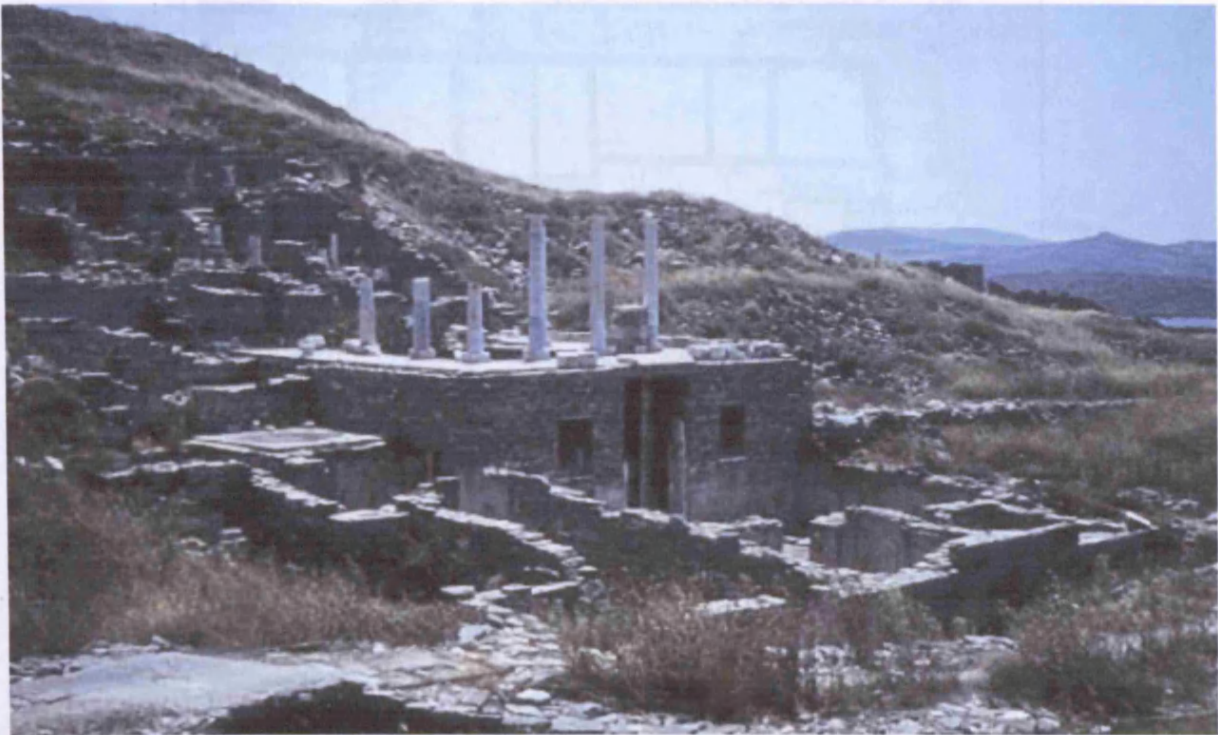
Figure 10. The House of Hermes (NE view). The concrete shelter served in the reconstruction of the 2 nd floor
