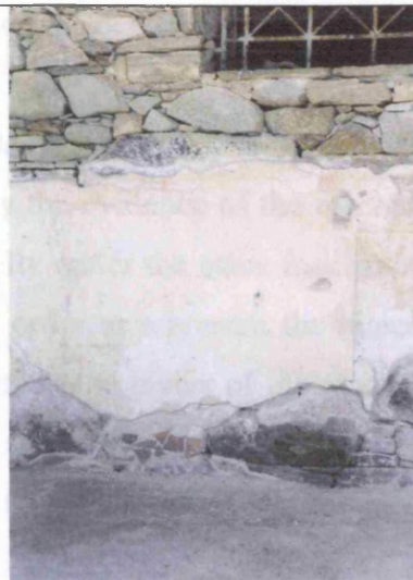
Figure 8.3. Room MA, north wall
