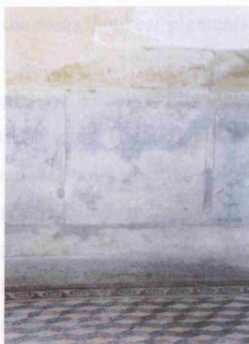
Figure 8.2. Room MD, north wall
