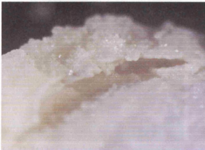
Fig. 28, 29 Lime wash large flakes detachment
