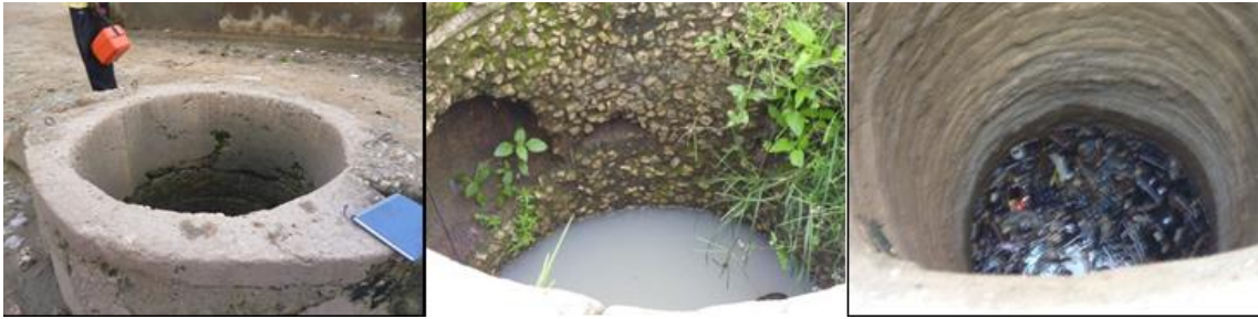
Figure 2.7: Polluted water due to refuse dump and natural vegetation growth in a typical dug well
