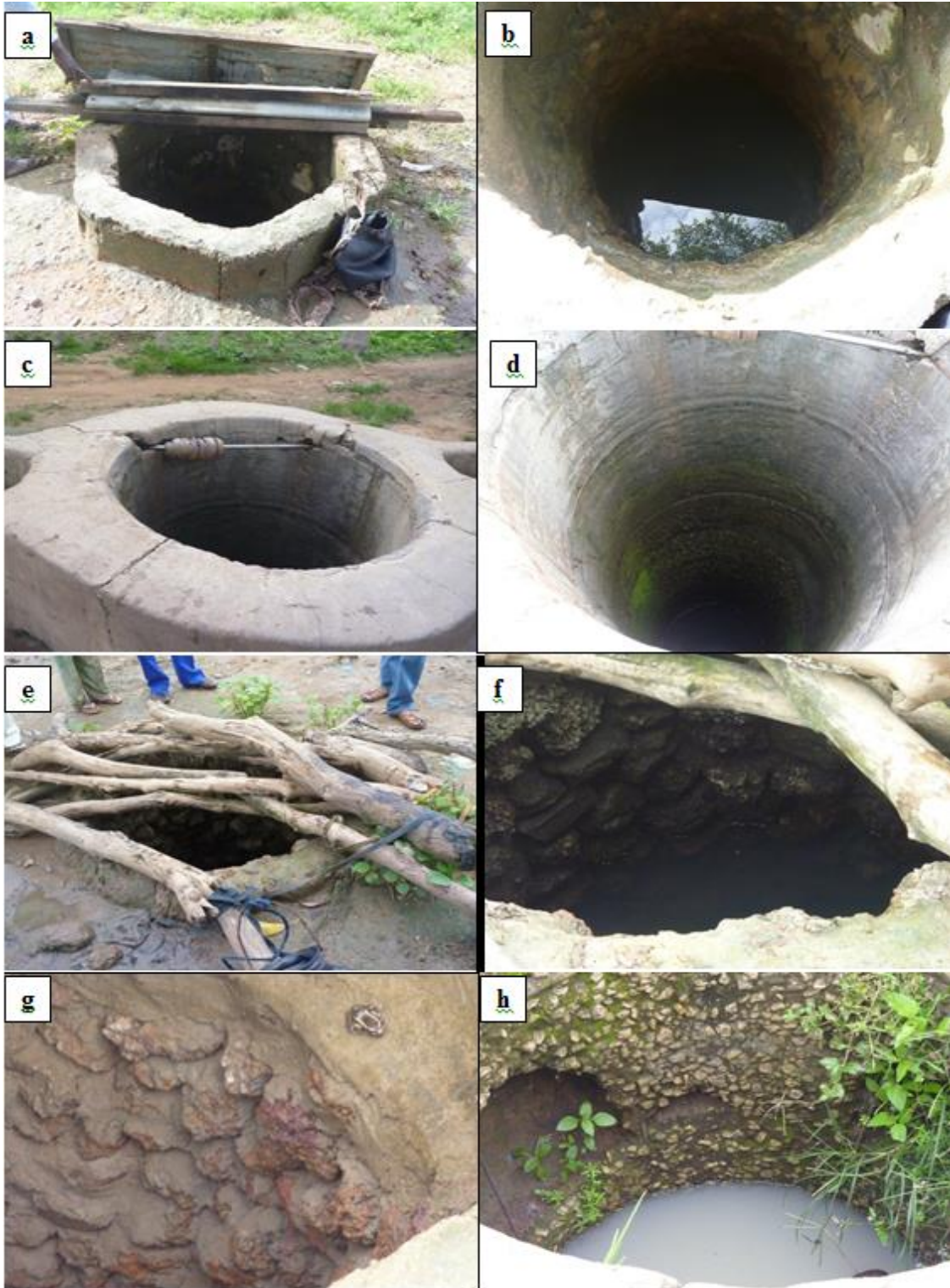
Figure 4.3: Pictures of hand dug wells in different locations in town landscape (a-b) shallow depth well with shallow water table and ‘guga’ used to withdraw the water; (c-d) deep hand dug well with deep water table and a raft across for water pulling; (e-f) shallow dug well in a house with water table close to the surface (within an arm-length); (g-h) shallow wells in town close to fadama usually of poor biological quality (note invasion of weeds and even frogs)
