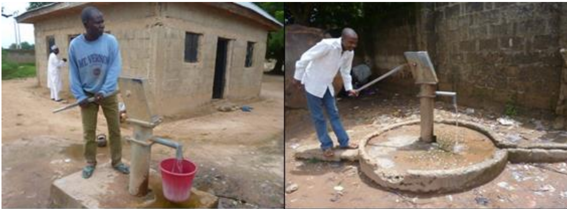
Figure 2.8: Typical hand pump boreholes found within the catchment
