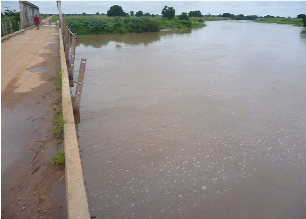
Figure 6.4: Photograph of Fokku Bridge with high flows in the River Ka
