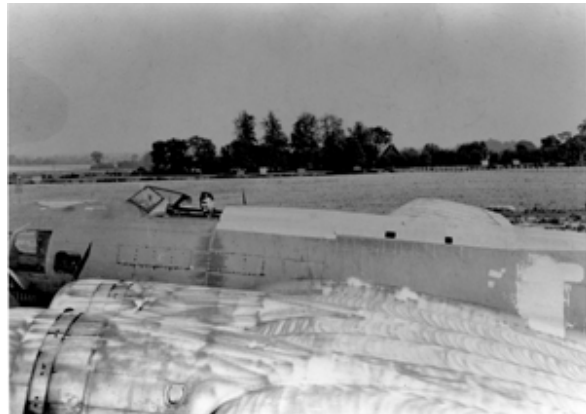
Figure 2.14: a pilot sitting in one of the stripped-down bombers used in Aphrodite project; once airborne the pilot bailed out from the plane. Source: [46]
