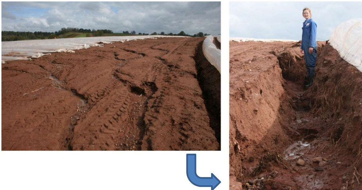
Figure 2.6. Gully formation from asparagus wheelings. Runoff from the compacted wheelings forms deep rills in the relatively less-compacted track way. These rills run downslope, and merge to form one deep gully.
