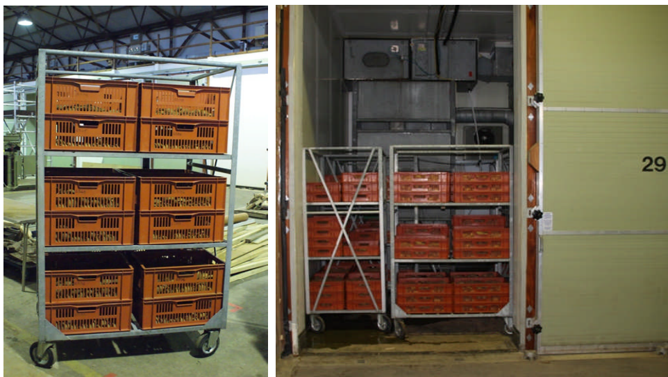
Figure 3.6 Storage of tubers in 10 Kg capacity trays into the specifically modified for ethylene store room
