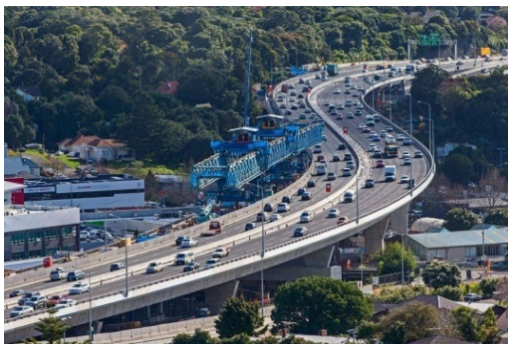
Figure 1. Aerial view of Newmarket Viaduct.
