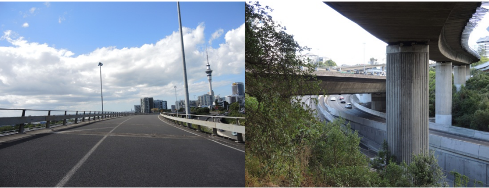
Figure 1. Views of the Nelson St off-ramp bridge
