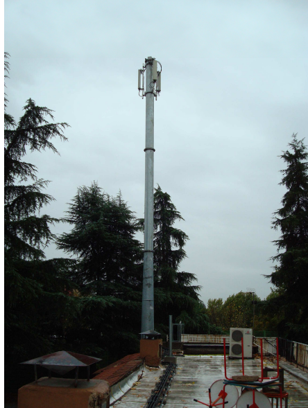
Fig 2.15 Torre monopolo o tubular 30 m
