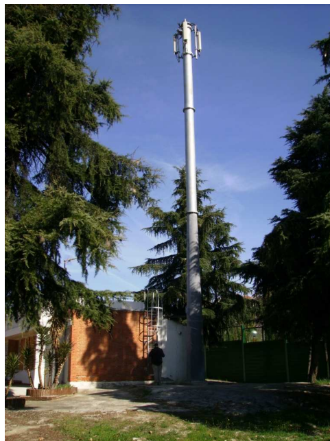
Fig 5.1 Torre tubular 20 m
