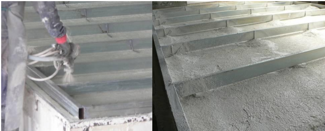
Fig. 2-6: Stud-frame typology: metallic frames are jointed to the GRC shells by projecting a dollop of GRC with a spray gun over the small pin attached to the trusses. The frame stiffens the shell for better bearing horizontal loads such as wind [DRA]
