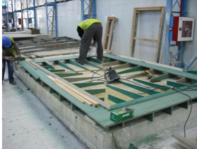
Fig. 4-9: Special moulds for conforming pyramidal shapes on panel P-10 [DRA-SEIS]
