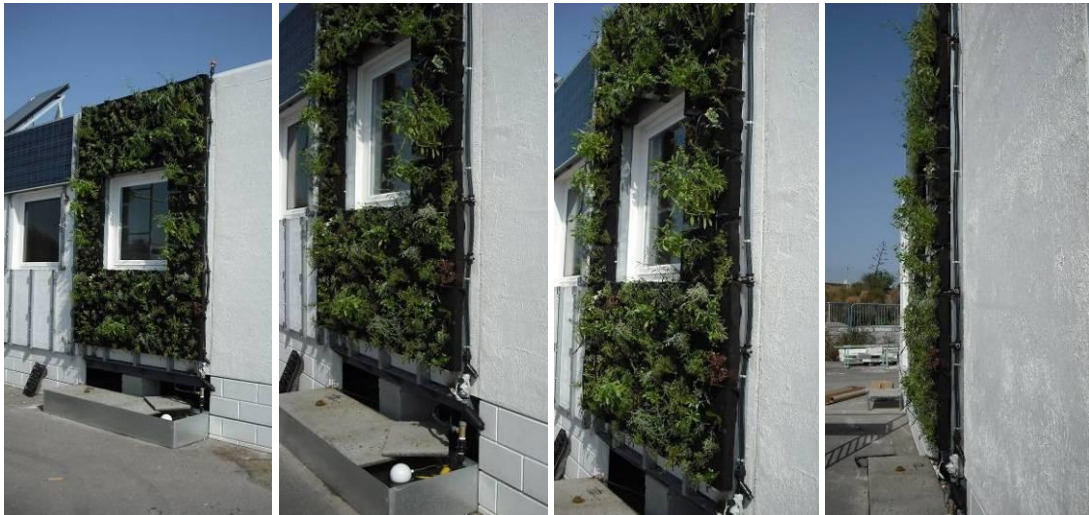
Fig. 4-16: Vegetated panels after installation onto Framex façade [DRA-SEIS]
