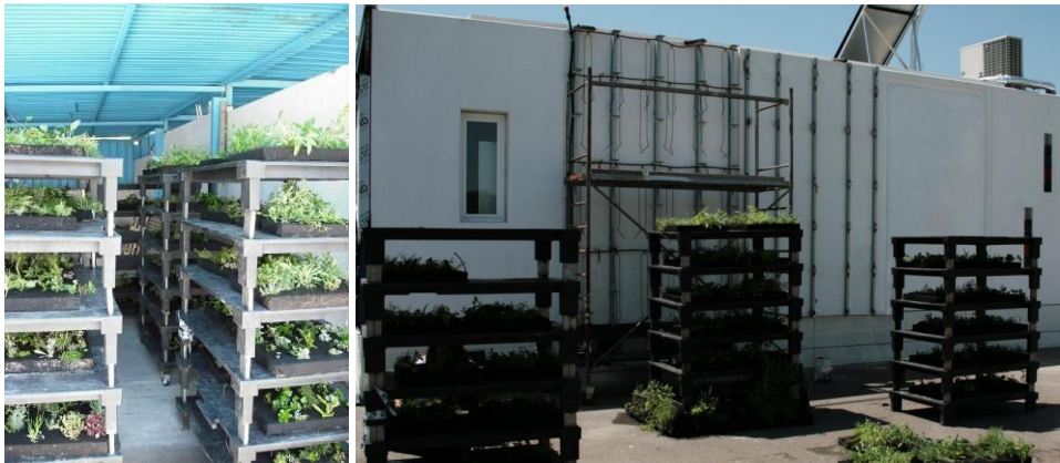
Fig. 4-13: Plants horizontally stocked for their better growing and align in front of façade P-08 prior to their installation [DRA-SEIS]
