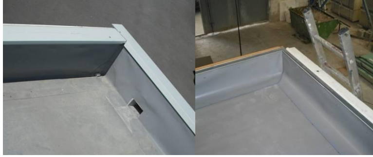
Fig. 4-8: Waterproofing membrane on the roof deck [DRA-SEIS]
