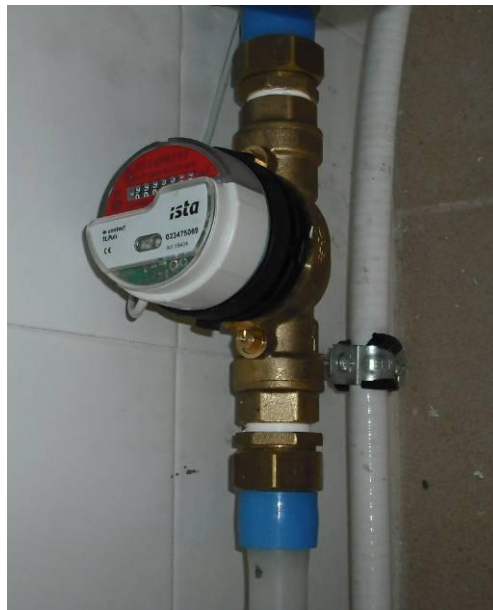
Fig. 3-5: Water meter installed in the Mock-up pipes [DRA]
