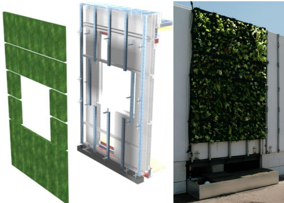
Fig. 4-14: Left, schematic of the vegetated cells lay-out and the Framex; Right, P-08 before completion: the underlying metallic profiles can be seen behind the green panels [DRA-SEIS]
