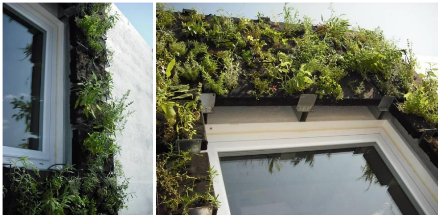
Fig. 4-17: Details of the vegetated panels around the window opening [DRA-SEIS]
