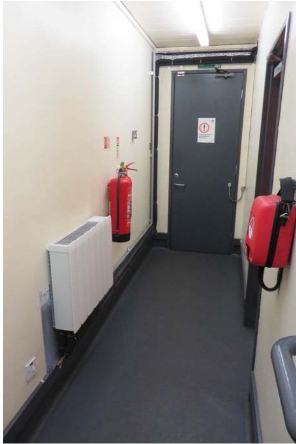
Figure 6: One of the four new radiators at the Station's corridor
