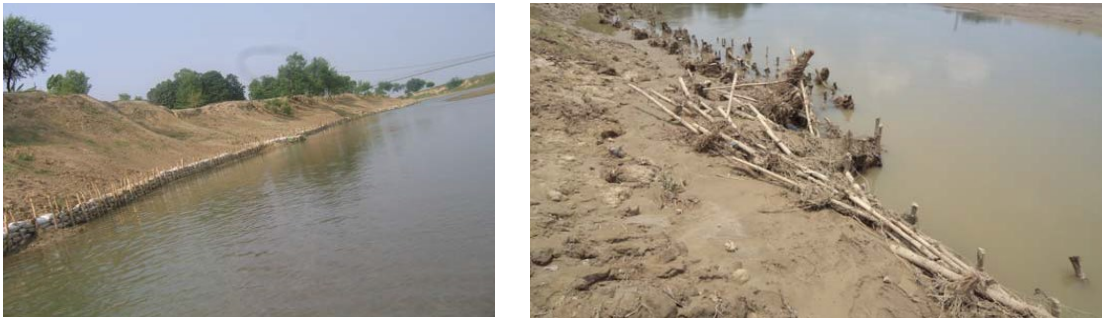
Figure X. Bamboo vanes and vetiver plantation a) before and b) after the flood event
