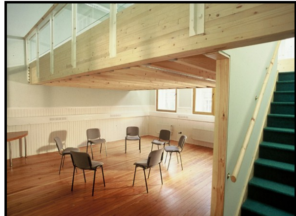
Figure 2: Mezzanines in Former Class Rooms
