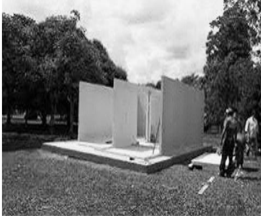
Figure 2.1 Polymer composite panels of floors and walls of houses (Inovatecsystem, 2006-2016)
