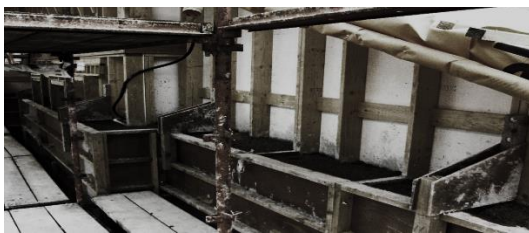
Figure 1.8 Hemp lime home under construction (Benhaim, 2013)
