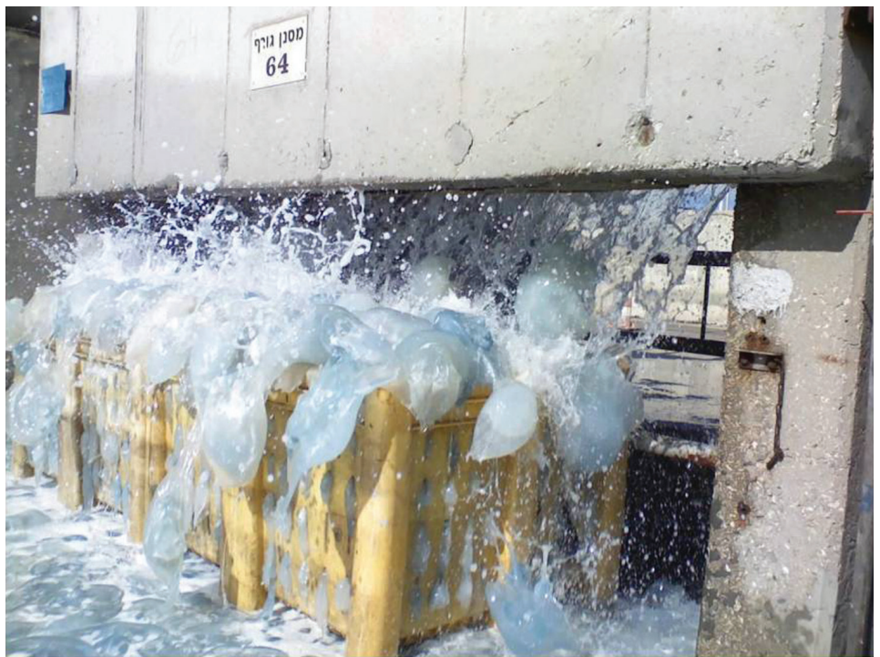
Fig. 3. A swarm of the scyphozoan jellyfish, Rhopilema nomadica , likely introduced through the Suez Canal, blocked water-intake pipes of power plant in Israel, 2011.
